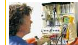
Insulation test at a distribution panel
